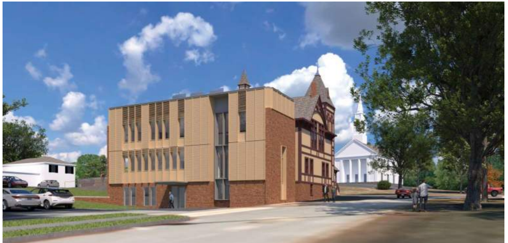
TOWN HALL ADDITION LOOKING NORTH
